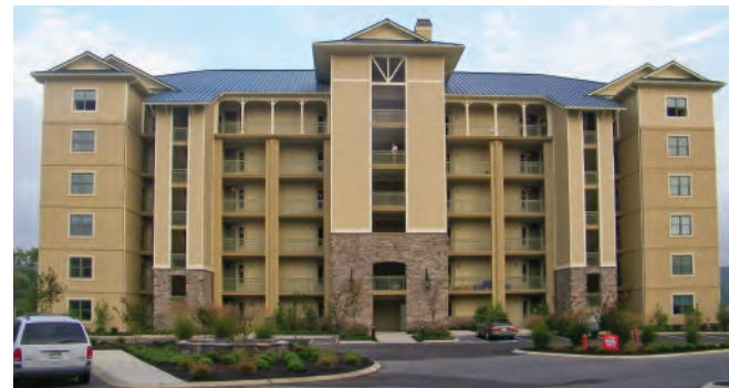
Waterside Tower Condo at Norris Lakes: ICF shell completed in 3 months
